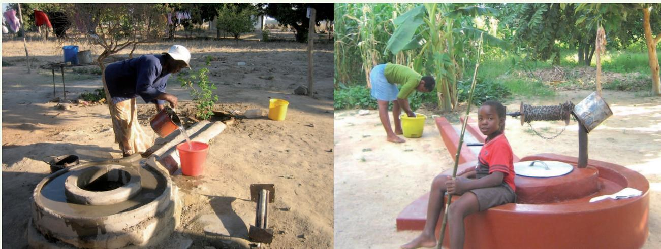
Figure 7: Left. A simple upgraded well built by the pupils. Right. The same well upgraded later with a windlass.
