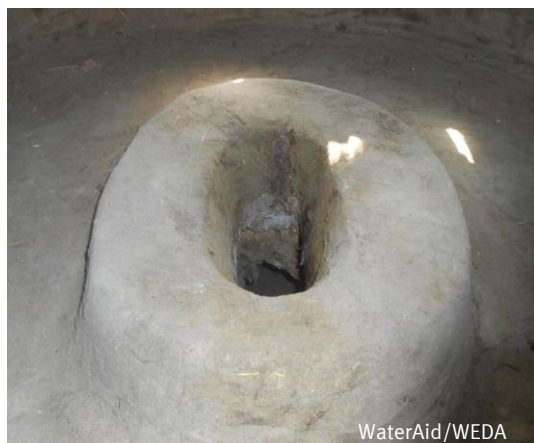
A fixed latrine seat made out of unburnt bricks smeared with local cement.
