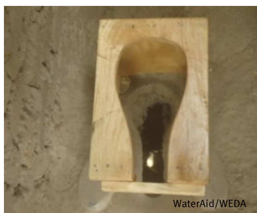
A moveable stool with a hole in the seat placed directly over the latrine drop hole.
