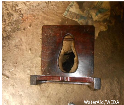
A moveable chair with a hole in the seat placed over the latrine drophole.
