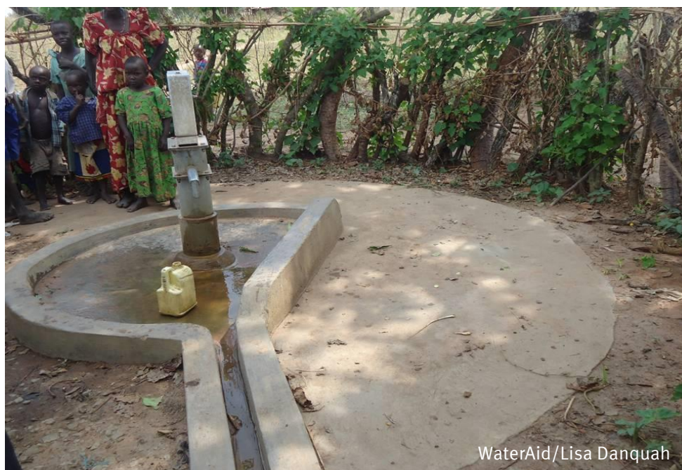
Inclusive apron design borehole by WEDA in the Omodai sub-county.
