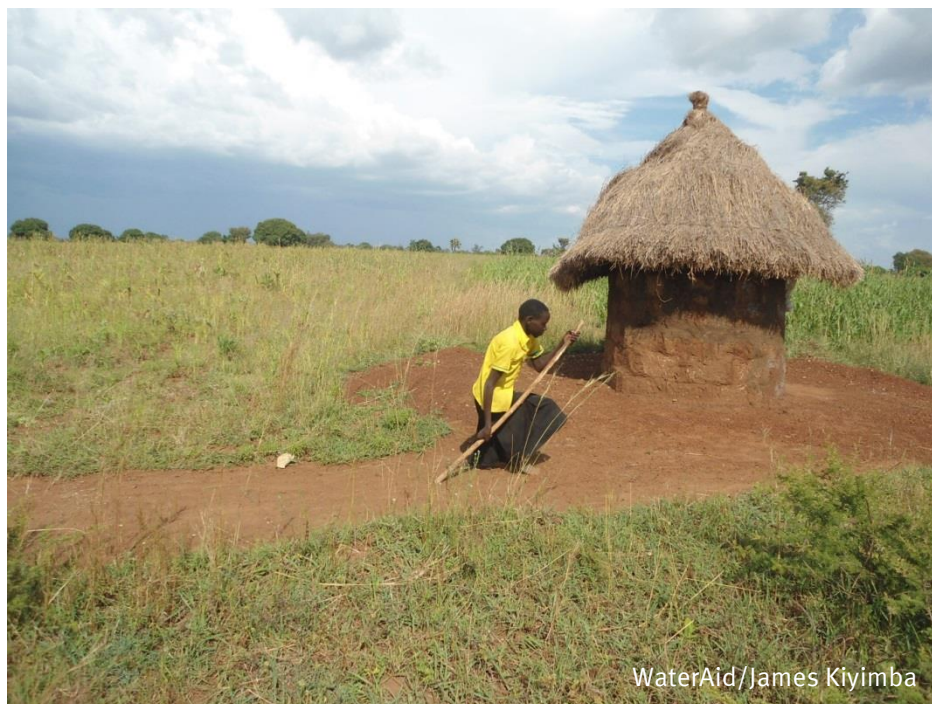
A levelled and cleared path to a household latrine.
