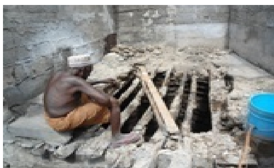
Photos 3 and 4. Preparation for manual pit emptying
