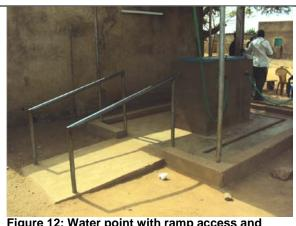
Figure 12: Water point with ramp access and handrails, Burkina Faso (Kpehounton and Serge 2012)
