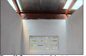
Figure 33: Transparent roof sheets to increase natural lighting (Badloe, 2012)
