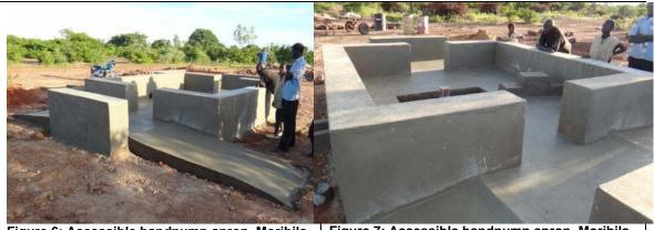
Figure 6: Accessible handpump apron, Moribila Ziékan, showing access ramp (World Vision Mali)
