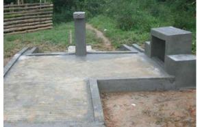
Figure 14: Water point apron under construction. Note laundry area and ramp access. (BESIK ndb)
