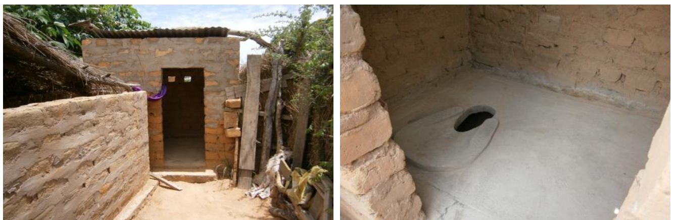
Figure 11: Improved pit latrine observed in one of the households in the surveyed wards
