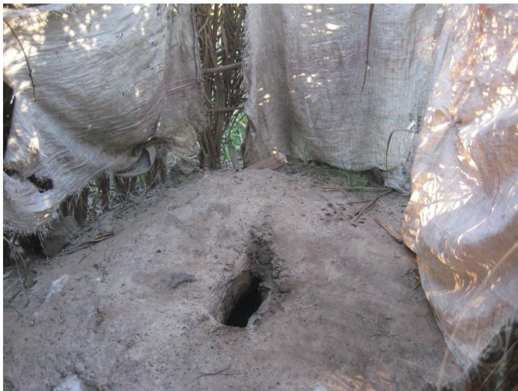
Figure 1. Un-improved sanitation: a simple pit latrine
