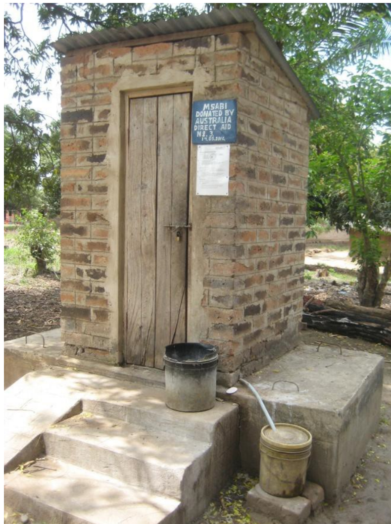
Figure 5. Improved sanitation – ecological sanitation with a double vault to compost sludge and urine diversion
