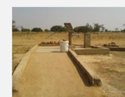
An accessible waterpoint in Zambia. It has a ramp, with raised sides to ensure wheelchair users don't fall off and which people with visual impairments can use as a guide. It also has a water bucket resting stand.
