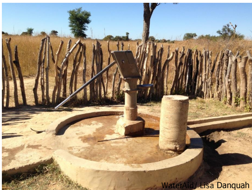
A waterpoint showing ramp and raised pedestal for water containers.
