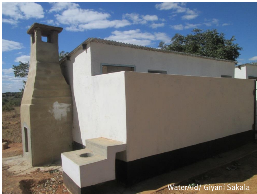
A newly installed school latrine block with an incinerator for burning menstrual waste and a handwashing stand in the foreground, Nkaba school.
